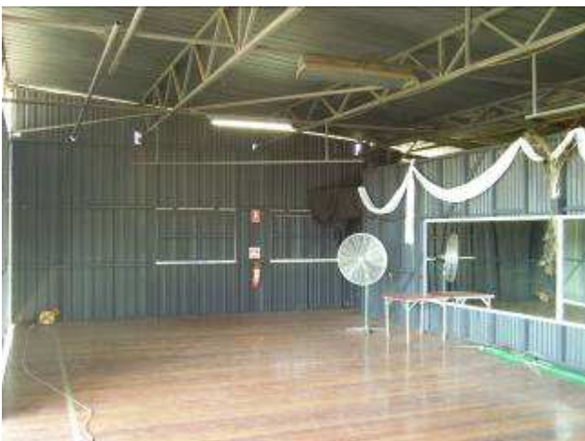
Stage right interior photo. Note upstage crossover wall with mirror, and diagonal scaffold bars in grid.
